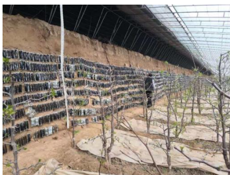
Fig.3. Winter jujube test base equipped with PCMs
